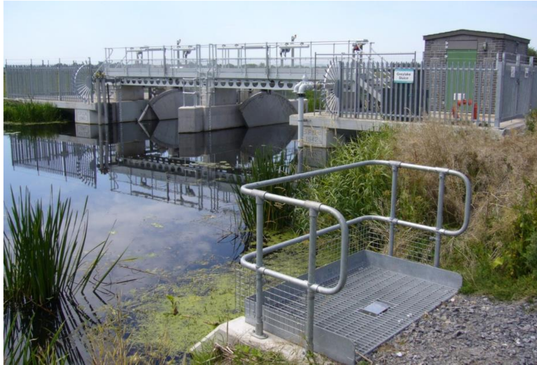
Greylake Sluice, King's Sedgemoor Drain: rebuilt 2005
